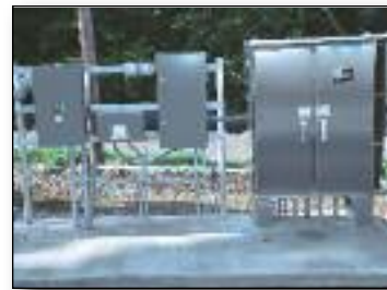
Shown clockwise from top left are the old Pitts Lift Station and wet well, upgrades to the Liberty and Pitts Lift Stations and a close look at the new electronic control panels installed for better operation of the stations.
